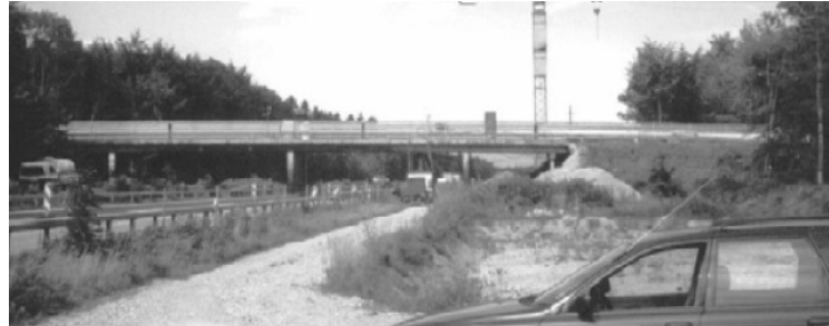
Z24 Bridge, Koppigen-Utzenstorf, Switzerland
